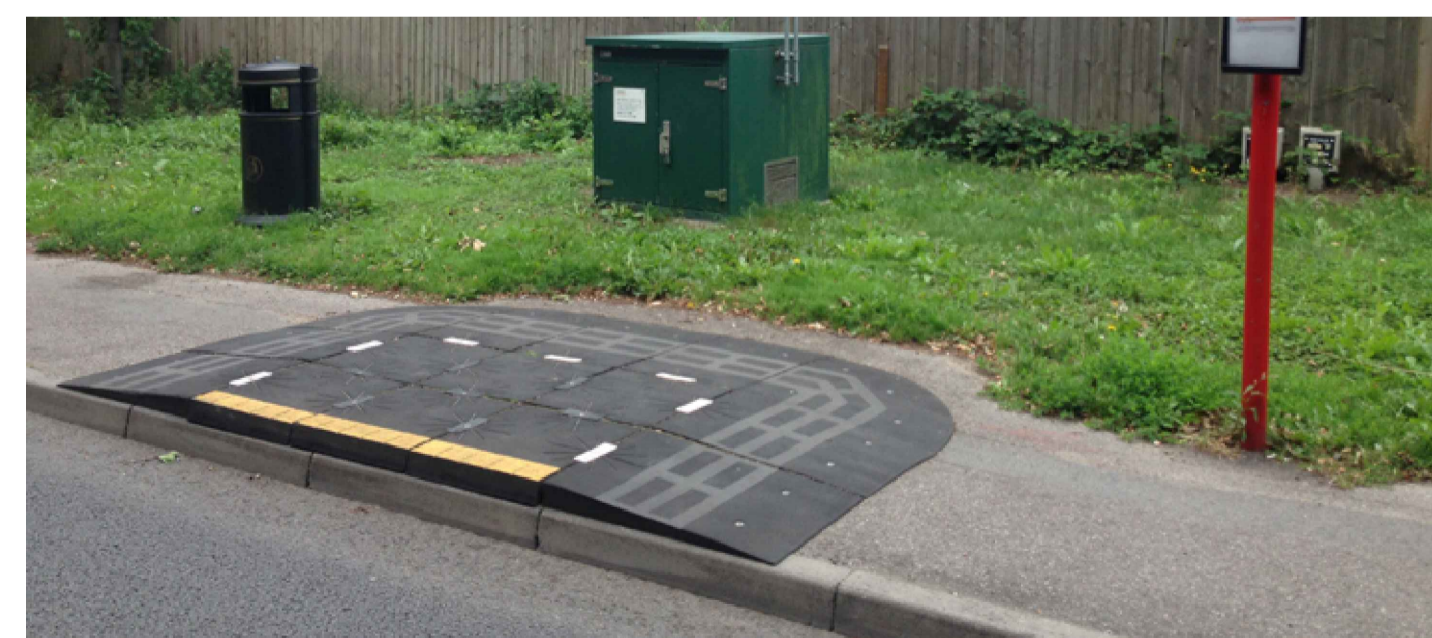
REDIWELD BUSPAD - TO BE LOCATED ON CARRIAGEWAY WHERE STATED SEE DRAWING COM-12727-1100-01 FOR CONSTRUCTION DETAILS http://www.rediweldtraffic.co.uk/products/inclusive-mobility/buspad/
