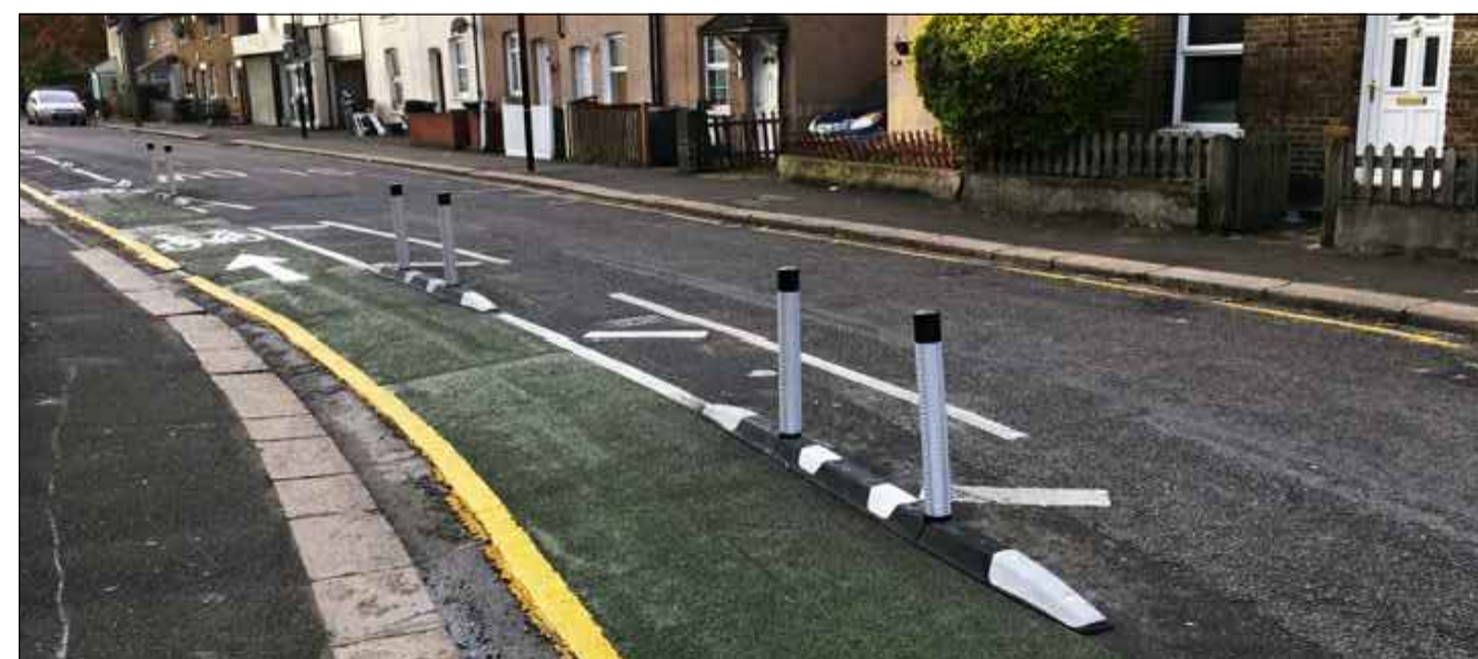
GREENWICH ORCA WANDS - 2.5m LONG SEE DRAWING COM-12727-1100-01 FOR CONSTRUCTION DETAILS http://www.rediweldtraffic.co.uk/products/cycle-lane-products/greenwich-wand-orca/
